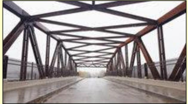
The new St. Anthony Parkway Bridge, which opened to traffic on October 27<sup>th</sup>, features a space-frame through-truss that references the historic Warren through-trusses of the original bridge.
