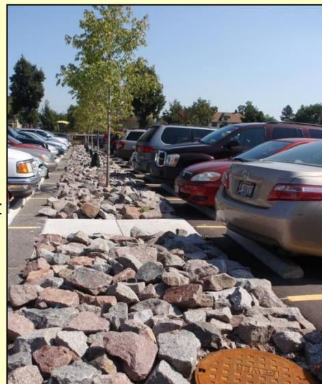
*A tree trench was installed in the renovated Edison High School parking lot. They absorb nutrients and filter runoff, helping to clean stormwater before it enters storm drains.
